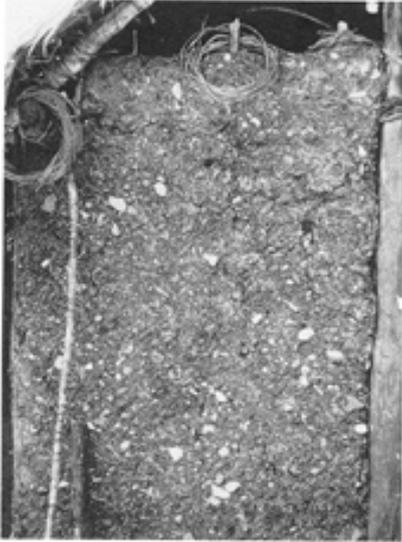
Fig. 5.6. A wattle-and-daub structure in Aguacatenango. Pottery sherds are often incorporated in the daub when it is excavated from previously occupied areas of the compound.
